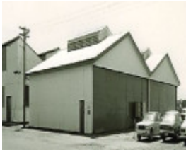
B4309 Building No 210
