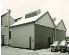
B4309 Building No 210
