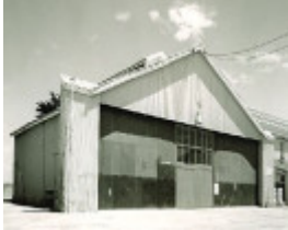
B4310 Building No 104
