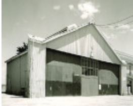
B4310 Building No 104
