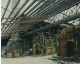
B6492 Wunderlich Terra Cotta Roof Tile Works
