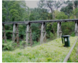
B2960 Puffing Billy Trestle Bridge
