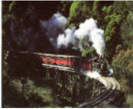
B2960 Puffing Billy Trestle Bridge
