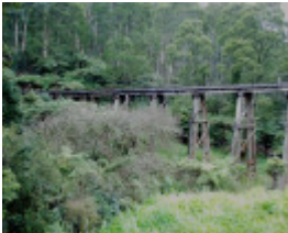
B2960 Puffing Billy Trestle Bridge
