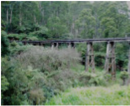
B2960 Puffing Billy Trestle Bridge
