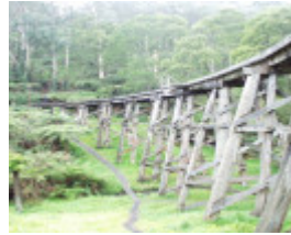
B2960 Puffing Billy Trestle Bridge
