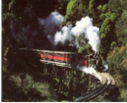
B2960 Puffing Billy Trestle Bridge
