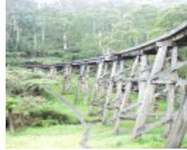
B2960 Puffing Billy Trestle Bridge
