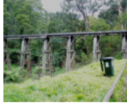
B2960 Puffing Billy Trestle Bridge
