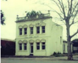
B5473 Former Colonial Bank
