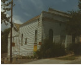
B5448 Former Mechanics Institute
