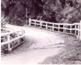
B7032 Myrtle Creek Bridge
