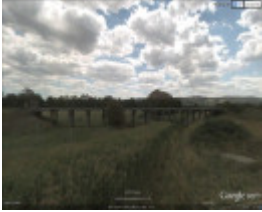
B7069 Stringybark Creek Bridge
