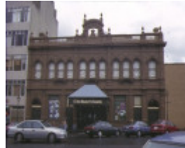
1 royal south street memorial theatre ballarat front view
