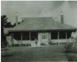
B2153 Mine Manager's Residence
