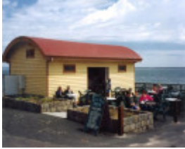
B6464 Jetty Shed
