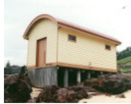
B6464 Jetty Shed
