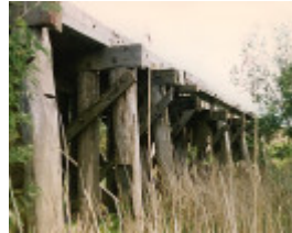
B6945 Lang Lang River Bridge
