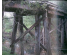
B6945 Lang Lang River Trestle Bridge
