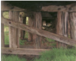
B6945 Lang Lang River Trestle Bridge
