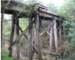
B6945 Lang Lang River Bridge
