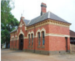
MALDON RAILWAY STATION COMPLEX SOHE 2008
