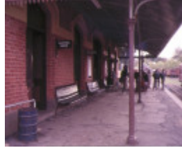
maldon railway station complex hornsby street maldon platform view
