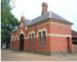
MALDON RAILWAY STATION COMPLEX SOHE 2008
