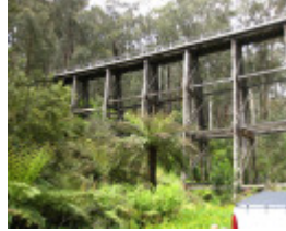
B1525 Noojee Rail trestle Bridge
