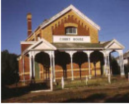
B3332 Wycheproof Court House
