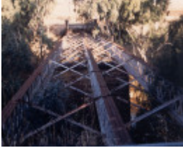
B7055 Glenmona Bridge
