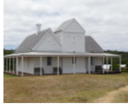
B2320 Cape Otway telegraph station
