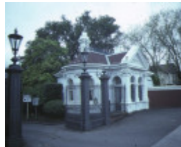
stonington glenferrie road malvern entrance gates sep1984
