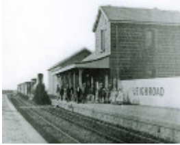
B2353 Railway Station Bannockburn
