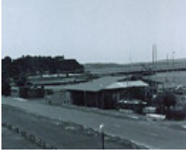
B6788 Former Railway Goods Shed
