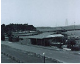
B6788 Former Railway Goods Shed
