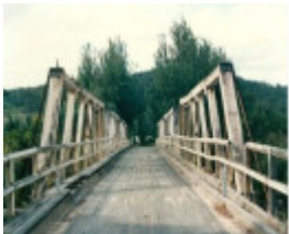
B2260 Genoa River Bridge
