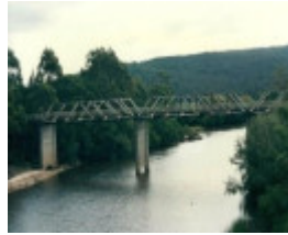
B2260 Genoa River Bridge
