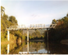
B2260 Genoa River Bridge
