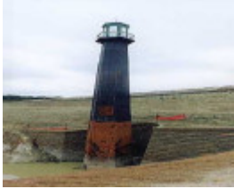
B7048 Outlet Tower
