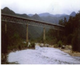
B6848 McKillops Bridge
