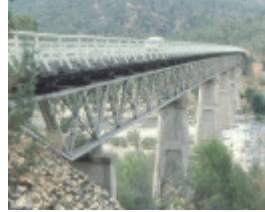
B6848 McKillops Bridge
