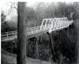
B6847 Murrindal Bridge
