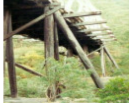
B6847 Murrindal Bridge
