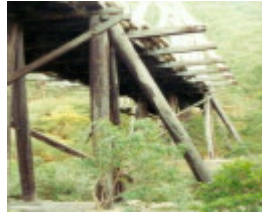
B6847 Murrindal Bridge
