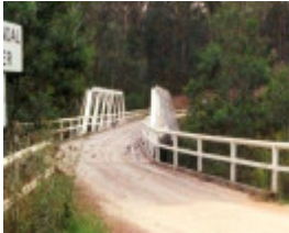
B6847 Murrindal Bridge
