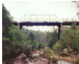
B6847 Murrindal Bridge
