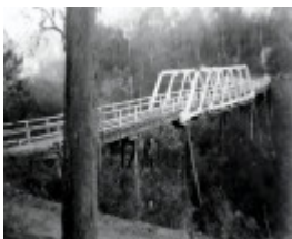
B6847 Murrindal Bridge
