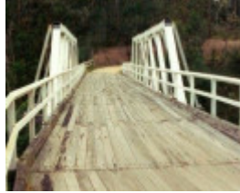
B6847 Murrindal Bridge
