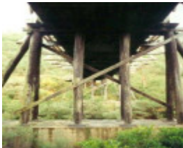
B6847 Murrindal Bridge
