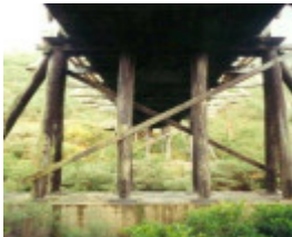
B6847 Murrindal Bridge
