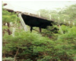
B6847 Murrindal Bridge
