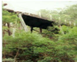
B6847 Murrindal Bridge
