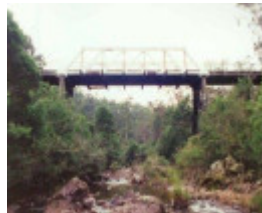
B6847 Murrindal Bridge
