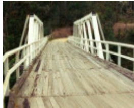
B6847 Murrindal Bridge
