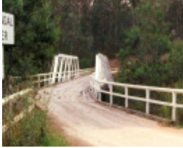
B6847 Murrindal Bridge
