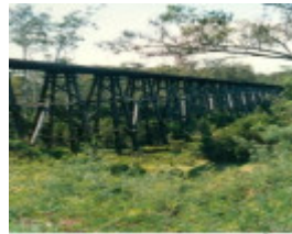
B3484 Stony Creek Bridge
