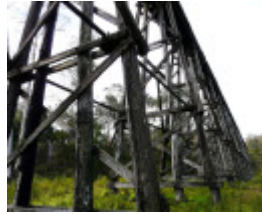
B3484 Stony Creek Bridge
