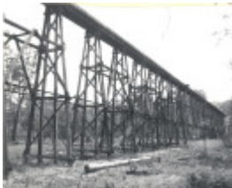
B3484 Stony Creek Bridge
