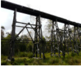
B3484 Stony Creek Bridge
