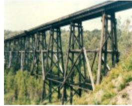
B3484 Stony Creek Bridge
