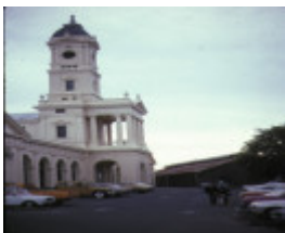
1 ballarat railway complex front view with tower feb1984
