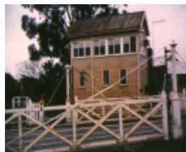
ballarat railway complex signal box & gates
