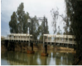
B4916 Barham-Koondrook Lift Bridge
