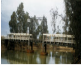
B4916 Barham-Koondrook Lift Bridge
