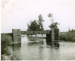
B2212 Hotspur Bridge
