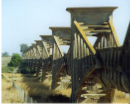
B5779 Ovoid Sewer Aqueduct
