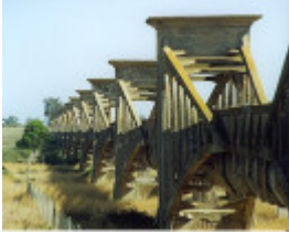
B5779 Ovoid Sewer Aqueduct
