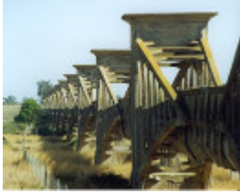
B5779 Ovoid Sewer Aqueduct
