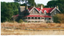
B1277 Elcho Homestead State significance (Vic. 01) State (Vic. 1881 to 1911) and (Commonwealth) (Vic. 1911 to 1970) and (Vic. 1970 to 1980) and (Vic. 1980 to 1981) and (Vic. 1981 to 1982) and (Vic. 1982 to 1983) and (Vic. 1983 to 1984) and (Vic. 1984 to 1985) and (Vic. 1985 to 1986) and (Vic. 1986 to 1987) and (Vic. 1987 to 1988) and (Vic. 1988 to 1989) and (Vic. 1989 to 1990) and (Vic. 1990 to 1991) and (Vic. 1991 to 1992) and (Vic. 1992 to 1993) and (Vic. 1993 to 1994) and (Vic. 1994 to 1995) and (Vic. 1995 to 1996) and (Vic. 1996 to 1997) and (Vic. 1997 to 1998) and (Vic. 1998 to 1999) and (Vic. 1999 to 2000) and (Vic. 2000 to 2001) and (Vic. 2001 to 2002) and (Vic. 2002 to 2003) and (Vic. 2003 to 2004) and (Vic. 2004 to 2005) and (Vic. 2005 to 2006) and (Vic. 2006 to 2007) and (Vic. 2007 to 2008) and (Vic. 2008 to 2009) and (Vic. 2009 to 2010) and (Vic. 2010 to 2011) and (Vic. 2011 to 2012) and (Vic. 2012 to 2013) and (Vic. 2013 to 2014) and (Vic. 2014 to 2015) and (Vic. 2015 to 2016) and (Vic. 2016 to 2017) and (Vic. 2017 to 2018) and (Vic. 2018 to 2019) and (Vic. 2019 to 2020) and (Vic. 2020 to 2021) and (Vic. 2021 to 2022) and (Vic. 2022 to 2023) and (Vic. 2023 to 2024) and (Vic. 2024 to 2025)
