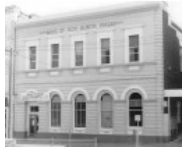
B3980 Fmr Bank of NSW View St Bendigo
