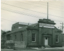
B3089 Former Waterworks & Sewerage Trust
