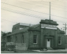
B3089 Former Waterworks & Sewerage Trust
