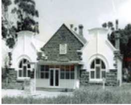
B1730 Old Shire Hall
