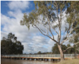
B7031 Murchison Rail Trail bridge 2010
