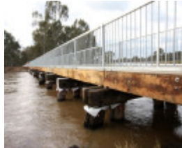
B7031 Murchison Rail Trail bridge 2010
