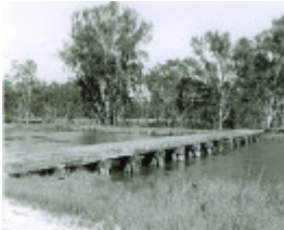
B7031 Murchison rail bridge
