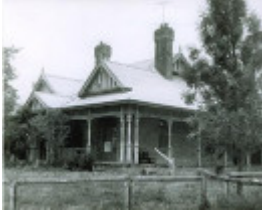
B3649 Old Wanganui Homestead
