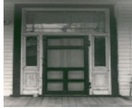
B1805 Rosebrook front Doorway
