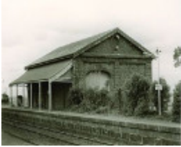
B5319 Goods Shed, Riddell's Creek station
