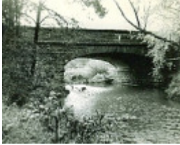
B0659 Woodend Bridge
