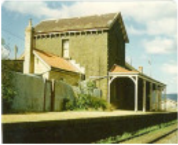
B4912 Railway Station Carlsruhe
