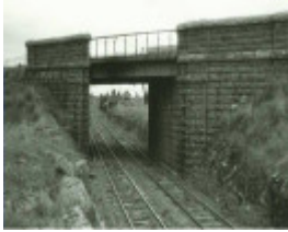
B7196 Bluestone Bridge
