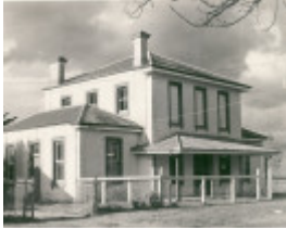
B2086 Former Court House & Police Station
