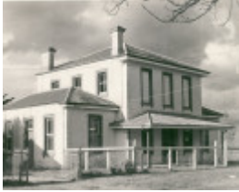
B2086 Former Court House & Police Station
