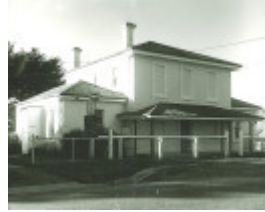
B2086 Former Court House & Police Station
