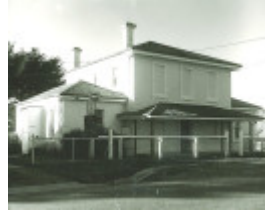
B2086 Former Court House & Police Station
