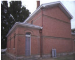
mansfield court house rear elevation feb1985
