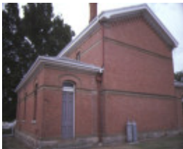
mansfield court house rear elevation feb1985
