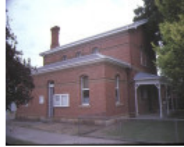
1 mansfield court house side elevation from front feb1985
