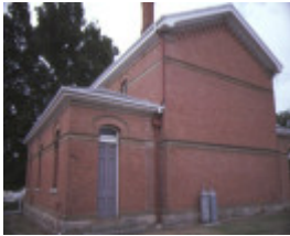
mansfield court house rear elevation feb1985
