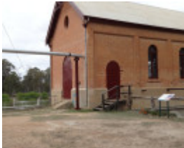
B3577 Psyche Bend pump house
