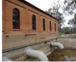
B3577 Psyche Bend pump house
