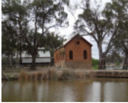
B3577 Psyche Bend pump house
