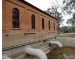
B3577 Psyche Bend pump house
