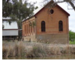
B3577 Psyche Bend pump house
