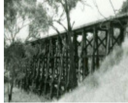
B3287 Railway Bridge Pyalong
