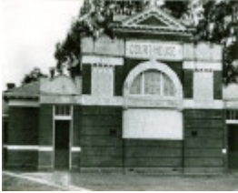
B3808 Fmr Court House Seymour
