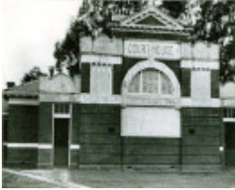
B3808 Fmr Court House Seymour
