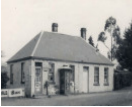
B0723 Former Post Office
