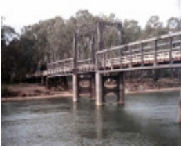
B6942 Cobram Bridge
