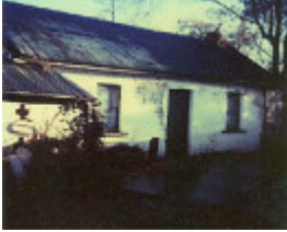
B5548 Ellerslie Cottage & Storeroom
