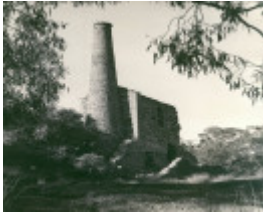
B1762 Ruins of Duke of Cornwall Mine
