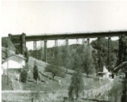
B1234 Railway Viaduct Taradale
