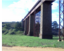
B1234 Taradale viaduct
