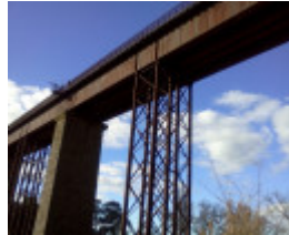
B1234 Taradale viaduct
